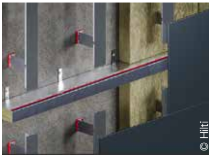
Fig. 1 left: Current fixture system for facade elements
